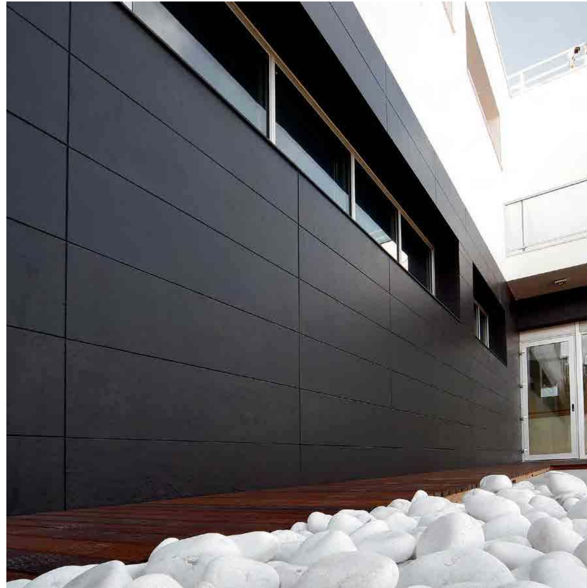
Seth Offices - Algés, Portugal - architect: BRUNO SERQUEIRA
